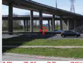
Infrastructure & Road construction
